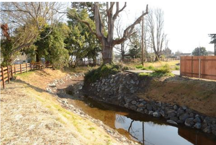
Image 16. Example Rock Slope Protection and Detail.
