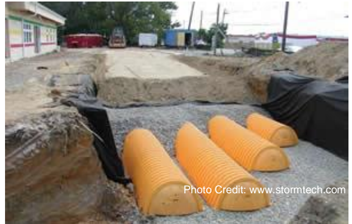
Image 8. Example Sub-surface Detention System
