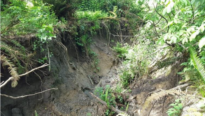
Image 9. Observed Channel Incision and Bank Failures
