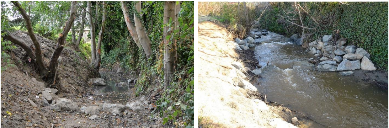
Image 11. Example Boulder Weirs Implemented to Arrest Channel Incision.
